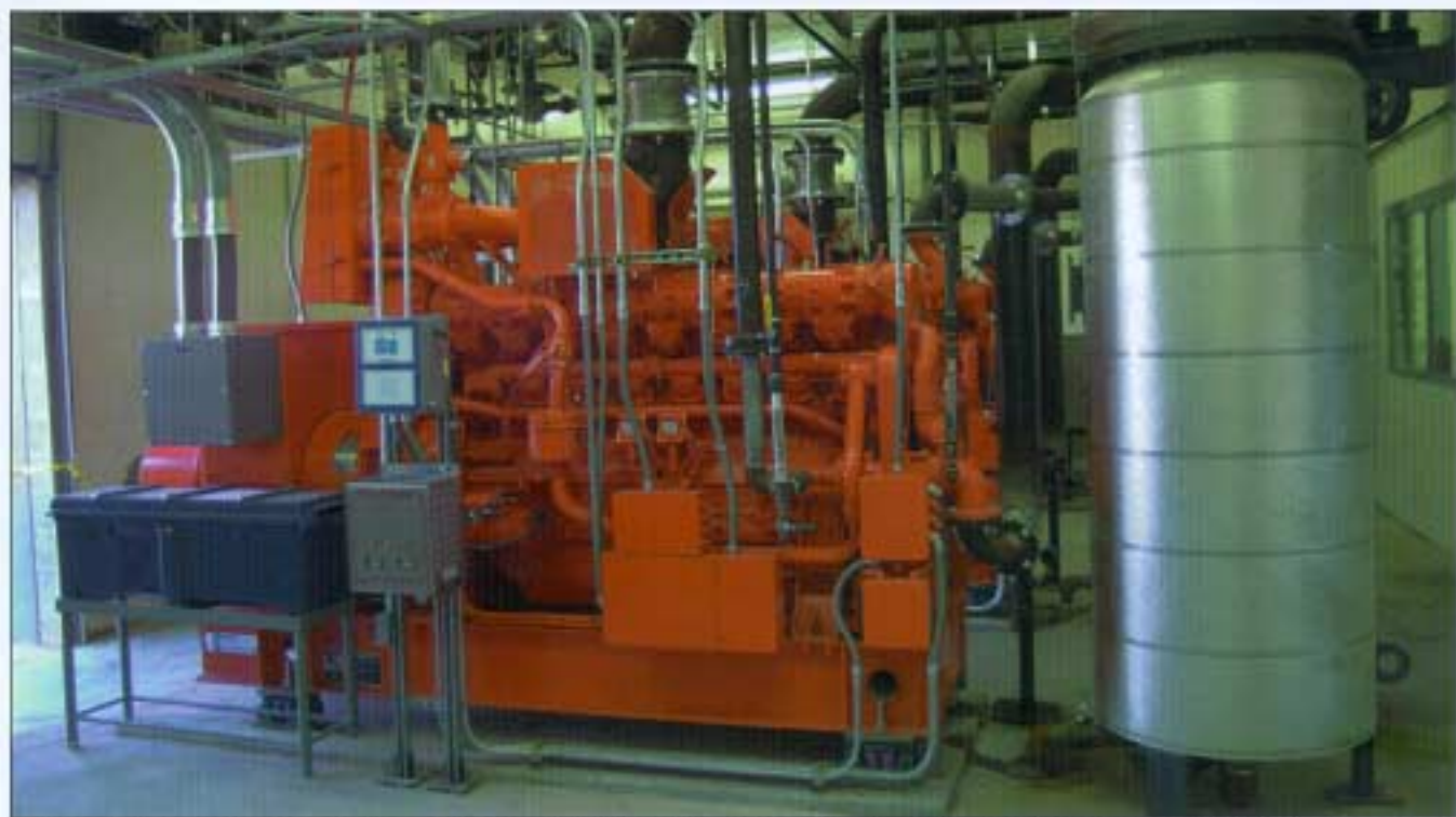
These two Waukesha Engine units use methane gas for fuel and provide more electricity than the farm uses and also provide hot water for the anaerobic sludge digestion which produces the methane. The extra energy is sold to the local utility at a profit.
